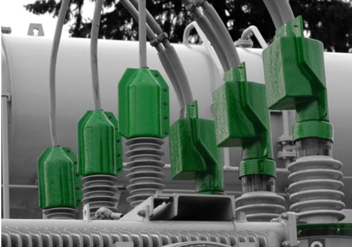
Installed on all our existing substations to prevent animal contact
