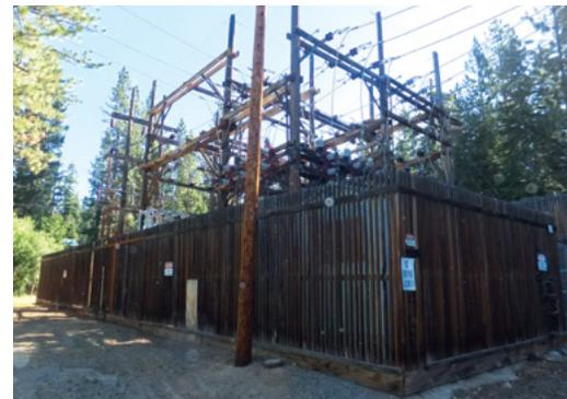
*The Brockway substation is about 50 years old and has reached the end of its useful life. Brockway experienced numerous problems during the winter storms earlier this year. Replacement and/or repair of existing parts are unfeasible and not cost effective.*
