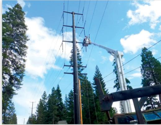
Known as the 650 Line Upgrade Project, this effort consisted mainly of replacing old wooden poles with those constructed of a brownish steel material that weathers with time to resemble wood as well as replacing wire to eventually operate at a higher voltage. The power line generally follows Hwy 267 from Truckee to Kings Beach.
