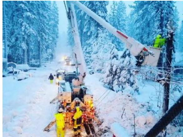
During the first week of storms, Liberty CalPeco’s system sustained outages on 15 of its circuits – affecting over 17,000 customers – due to falling trees and downed wires. Outages caused by falling trees and downed wires continued during the following weeks of the storms, impacting thousands of customers. The loss of three power sources into North Lake Tahoe caused by mud slides and falling trees during the second week of the storms impacted 22,000 customers.
