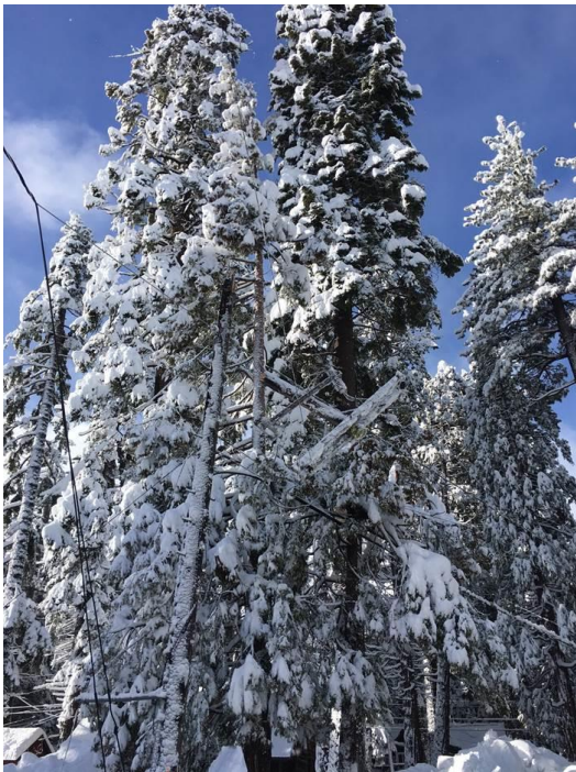
This broken power pole during the 2017 winter storms is difficult to see given the heavy snow and tree coverage.
